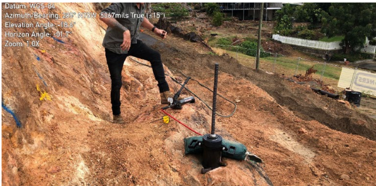
Figure 3 - On-site anchor pull-out test
