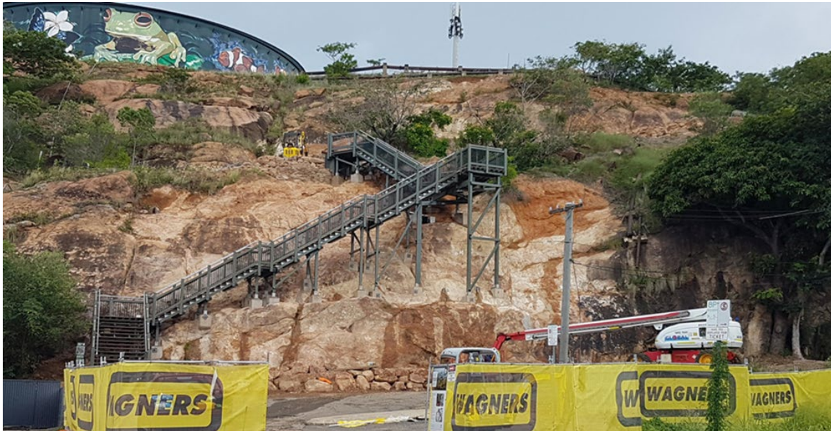
Figure 4 - Installed Castle Hills Stairs
