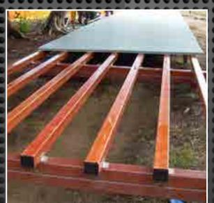
Wagners innovative boardwalk design allows composite structural members to be integrated with any type of pier, decking or handrail systems, including timber or steel. Composite boardwalk structures are easily assembled from fibre reinforced polymer (FRP) systems manufactured from FRP pultrusion structural shapes and composite sections.
