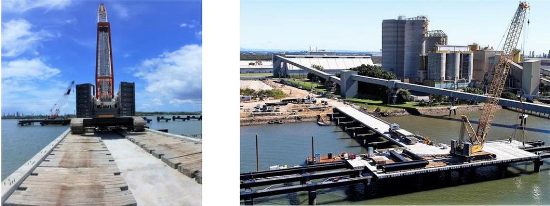
**Fig. 8** Mobile crane tracking on the wharf deck during construction
