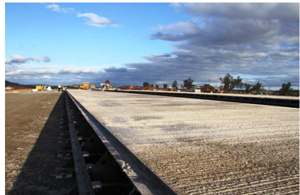
Figure 3: Curing and side forms with dowels.
