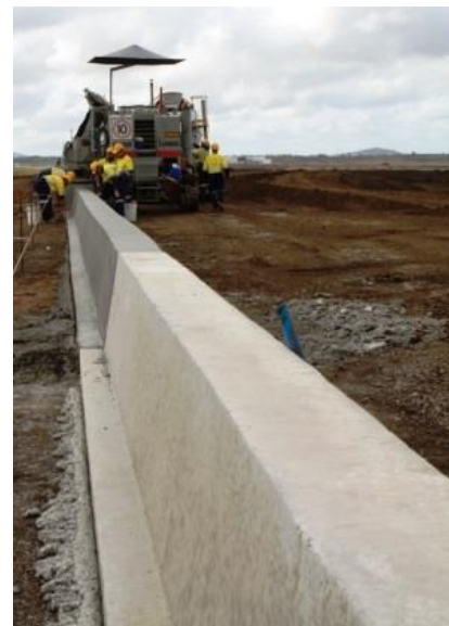
Figure 4. Other geopolymer concrete works at BWWA.
