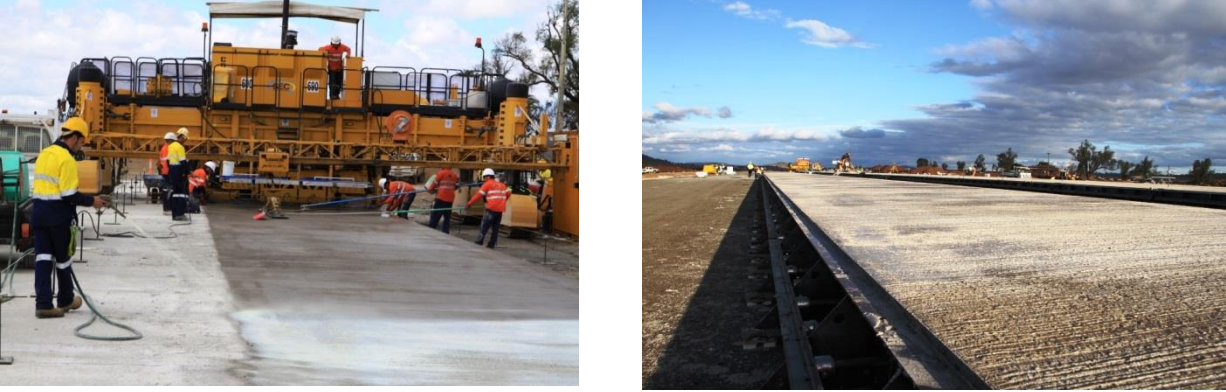
Figure 11. Curing and side forms with dowels.
