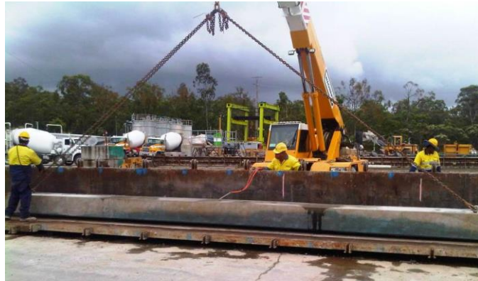
Beam de-moulding
