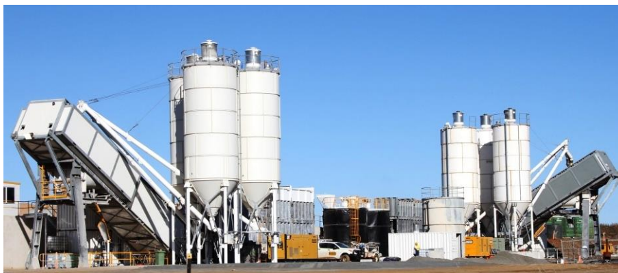
Figure 9. EFC twin batch plant.
