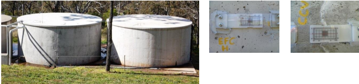
Figure 4 EFC Water Tank
