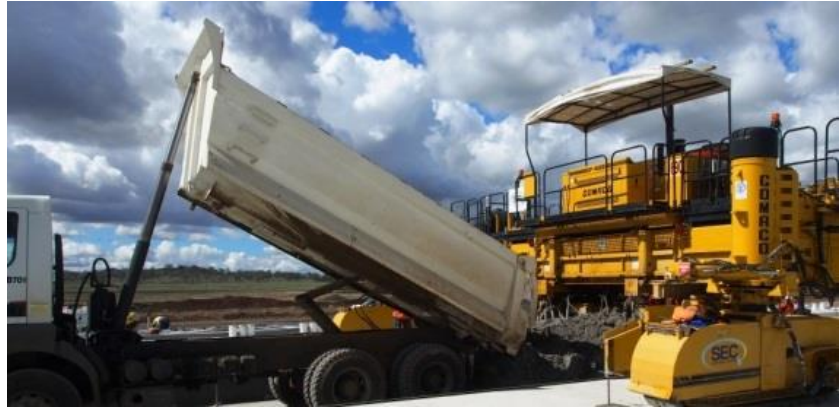
Figure 10. EFC delivery to slip form paver.
