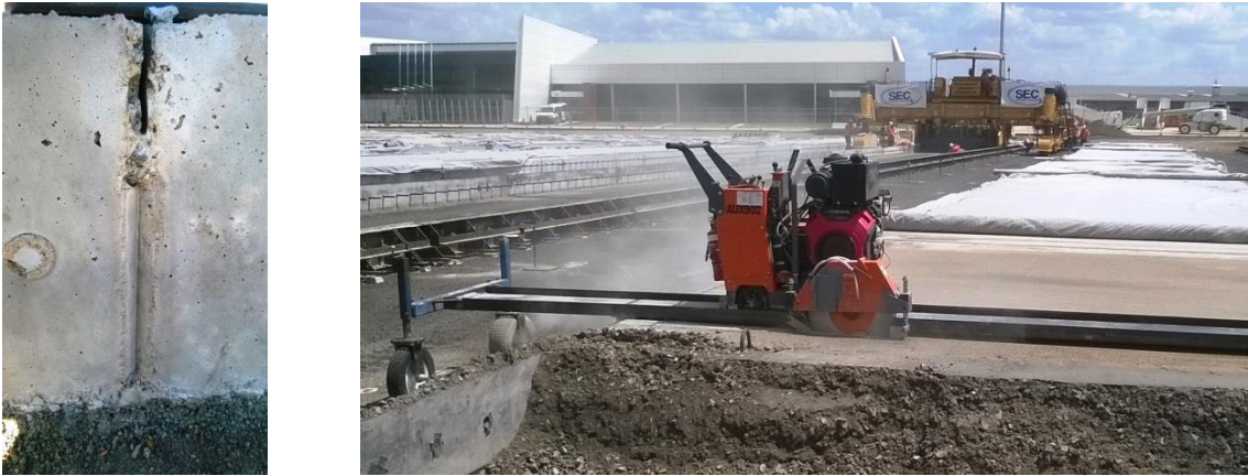
Fine crack in saw cut joint
