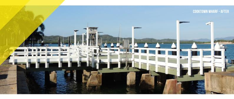
At times, rehabilitation rather than complete replacement of an asset is more appropriate. To ensure safety and longevity of a rehabilitated asset, Wagners have developed a timber replacement system. The system can either replace damaged and deteriorated timber components or provide a complete overhaul of the whole structure.
