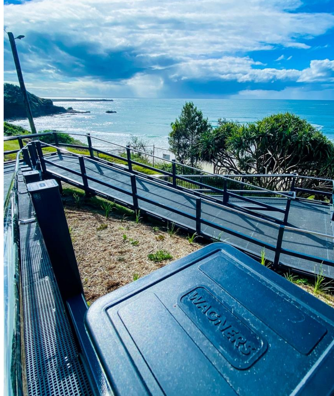
Upgrade to the zig-zag path in Yamba, NSW using Wagner's CFT
