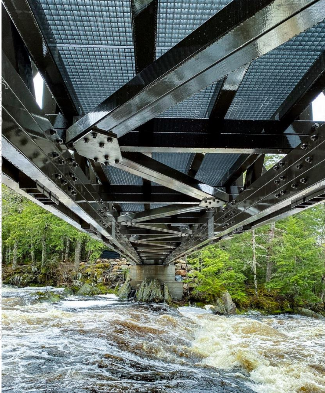
CFT Mersey River Bridge in Kejimikujik National Park, Nova Scotia, Canada
