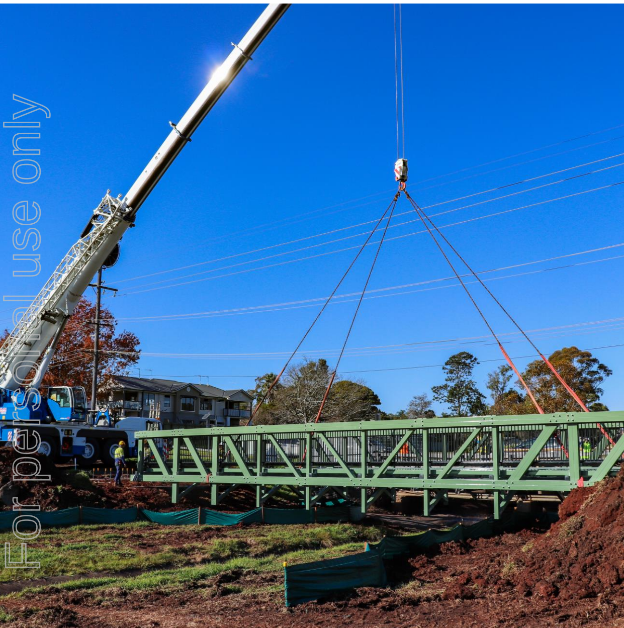
Alderley Street bridge installation in Toowoomba, QLD
