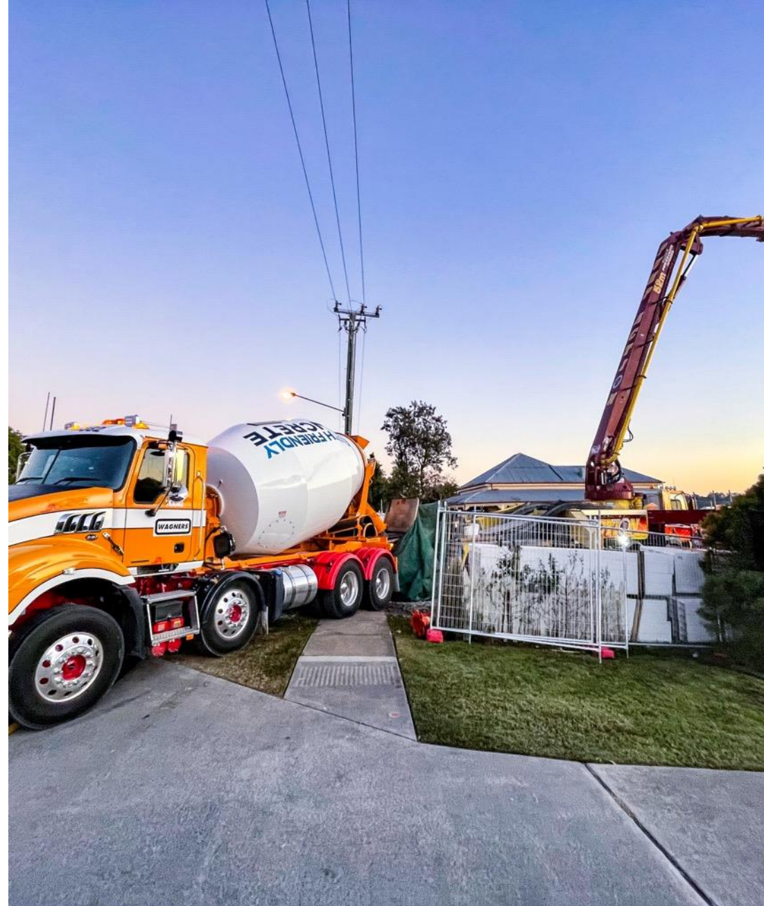
Earth Friendly Concrete® pour at Seventeen Mile Rocks, Brisbane
